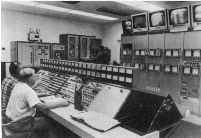
FIGURE 21-3. Control room (inside a reinforced concrete blockhouse) for test operators, instrument recorders, and controls. Note the control console, closed-circuit television, radio and telephone, direct read-out meters, strip charts, high-speed tape recorders, oscilloscope, air-quality alarm, and emergency lights. (Courtesy of U.S. Air Force Phillips Laboratory.)
